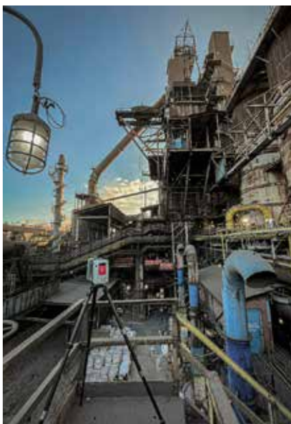
Fig.6. Scanning survey of a steel mill.
