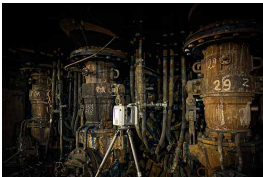
Fig.4. Scanning of the facility.
